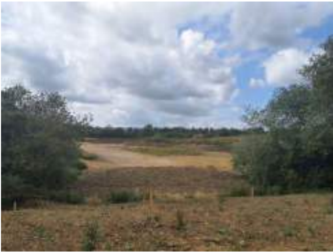
Figure 4.280: SWL1-1 – View from Beaufort Boulevard looking north into ongoing construction within the site.
