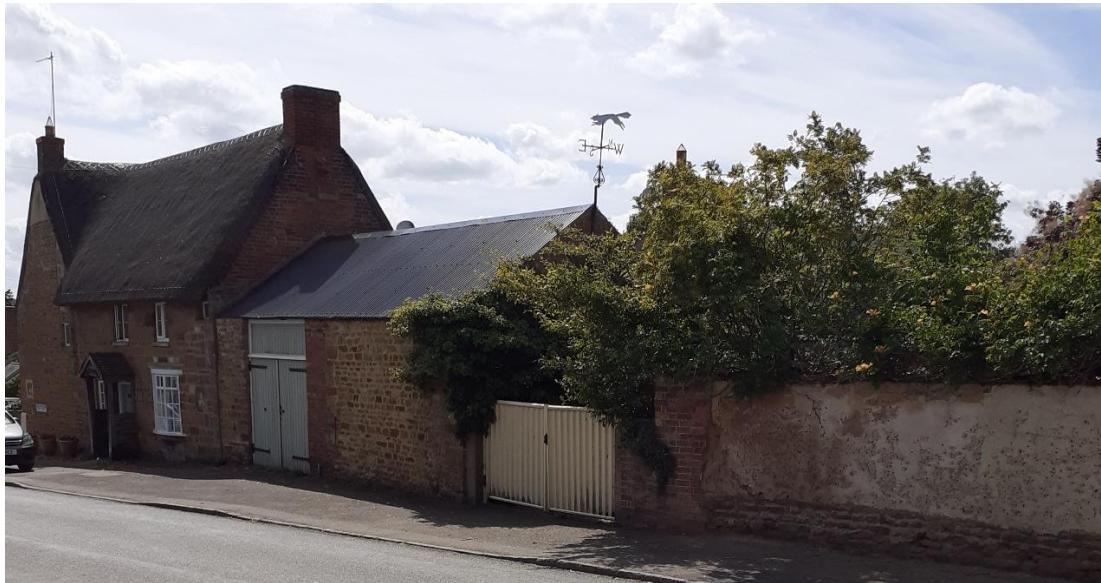
Fig.10. Stretch of mud wall on High Street.
