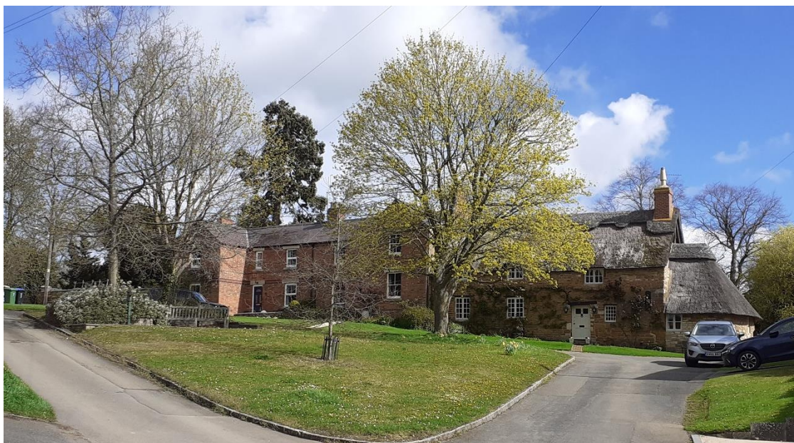
Fig. 9. View of the green on Church Bank with the water pump and seating area. 6 Church Bank can be seen behind the green to the right of the image.
