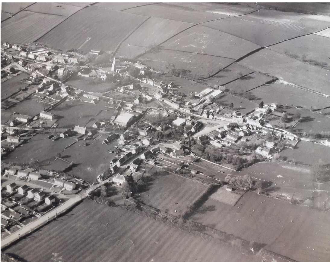
Fig. 4. Aerial view taken in the 1960s from outside the southern boundary of the conservation area on Barnsdale (Great Easton & District Local History Society Archive).
