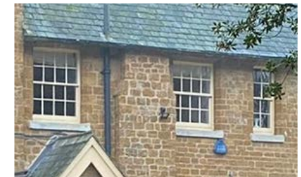
Georgian sash windows with wooden framing.
