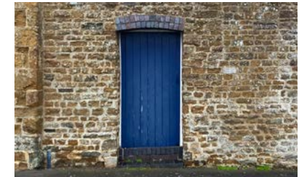
Simple wooden door with arched brick capping.
