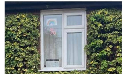
Three part casement window.
