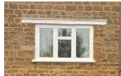
Rectangular casement window with long capping.
