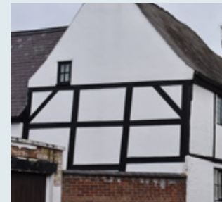
Timber frame with render over brick infill
