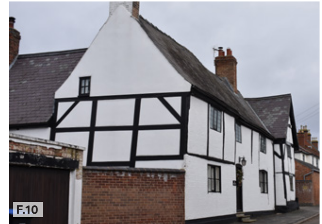
Figure 10: The Walnuts, which dates to the late 16th century. Timber frame with brick panel infill and Welsh slate roof. An impressive example of Tudor domestic architecture.
