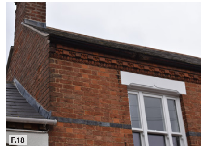
Figure 18: Example of detailed facade which creates visual interest on the street, with simple use of different coloured brick and ornament.
