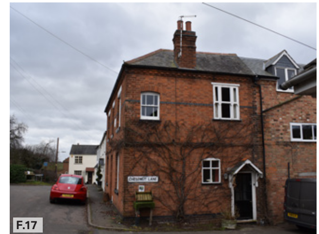
Figure 17: Example of a building with ornate architectural details and asymmetrical fenestrations, Chestnut Lane.
