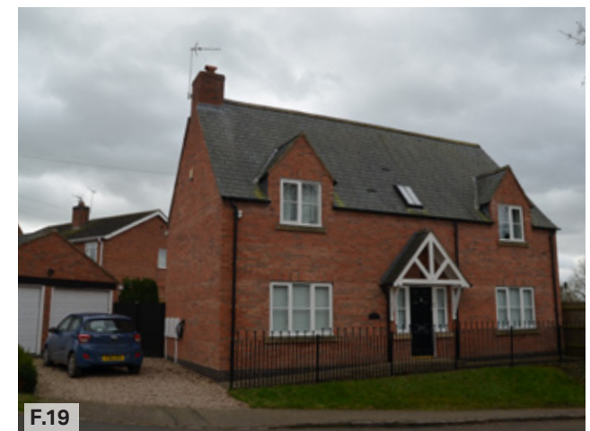
Figure 19: Example of on-plot parking to the side of dwelling.
