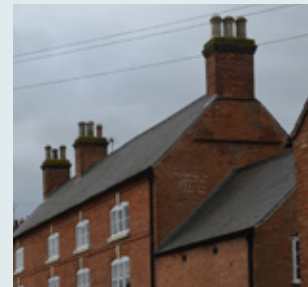
Chimney and decorative gable end
