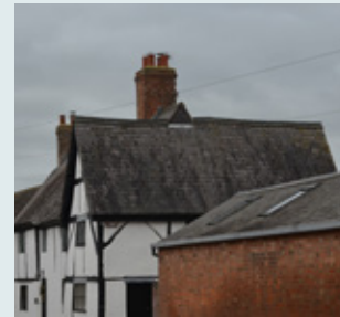
Varied roofscape and pitched roofs of different angles
